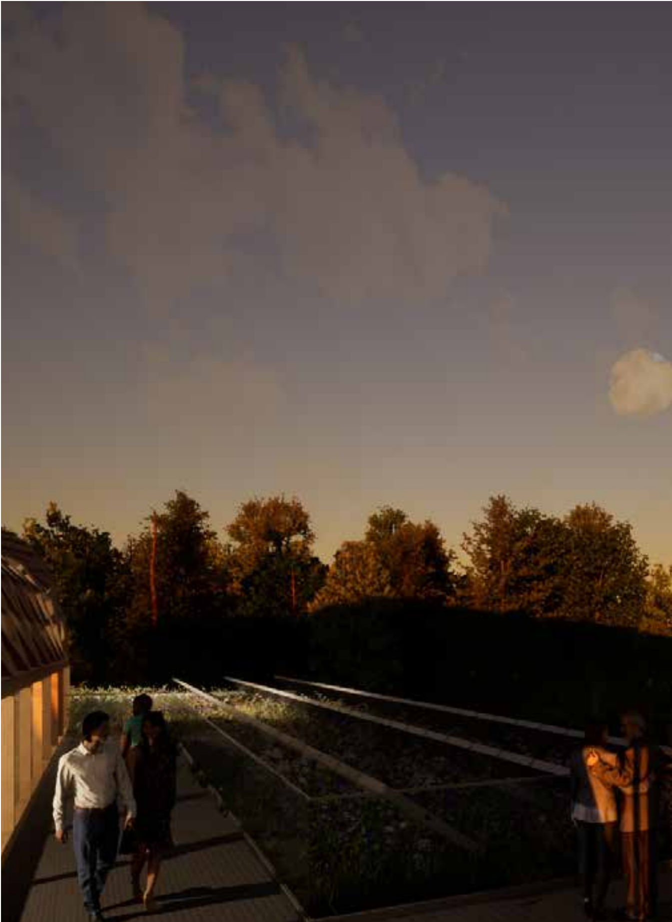
Figure 1. Night view of the roof top healing garden at the Athabasca Cultural Community Centre.
