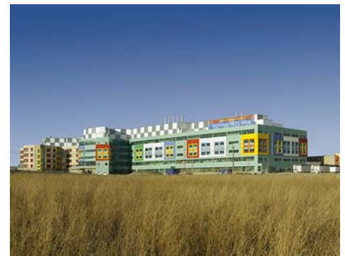
Alberta Children’s Hospital | photo: Robert Lemermeyer
