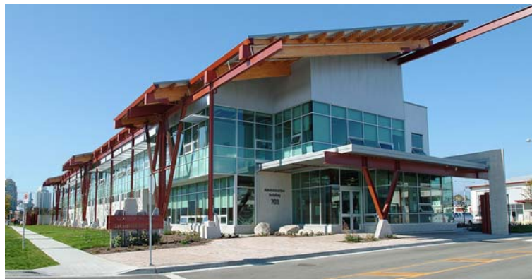
City of Vancouver National Works Yard, Certified CaGBC LEED 2.1 Gold | Omicron Architecture Engineering Construction Ltd. | photo: Terry Guscott
