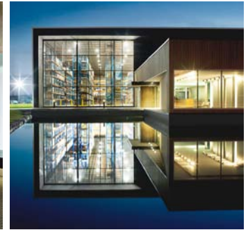
St-Germain Aqueducts and Sewers | photo: Marc Cramer
