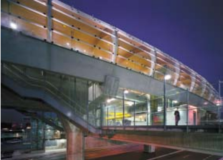
Brentwood SkyTrain Station / Busby + Associates Architects – Photo: Nic Lehoux
